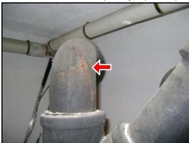
6.0 Picture 1 Cast iron waste line in basement.
